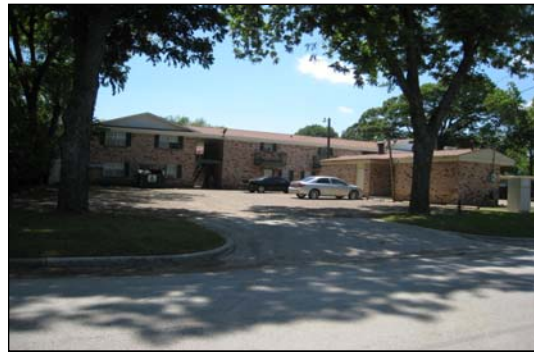
Rear Parking, Laundry, & Office
